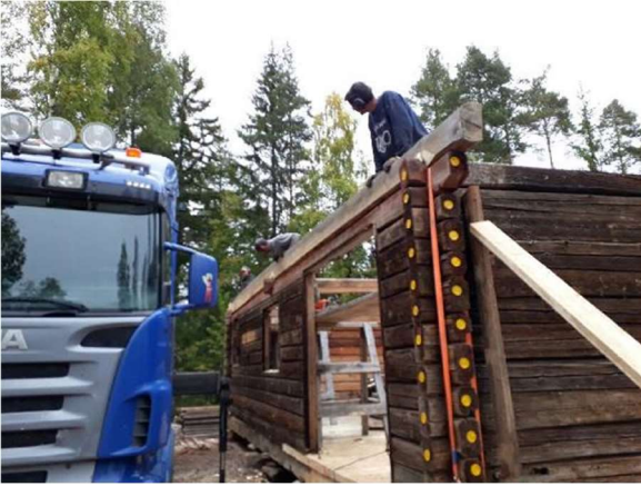
Ny stock under montering.
